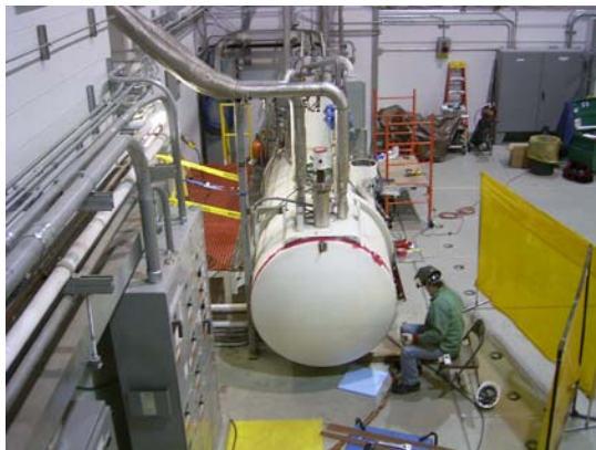
On-site Field Repair
