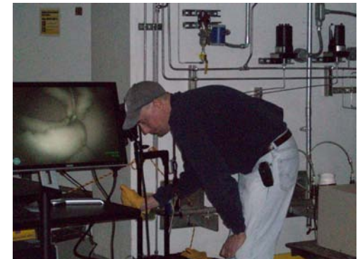
On-site VJ Line Remediation
