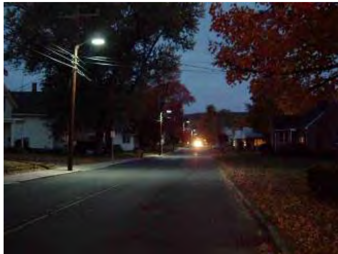
Figure A4-2. Fluorescent lighting with flat lens
