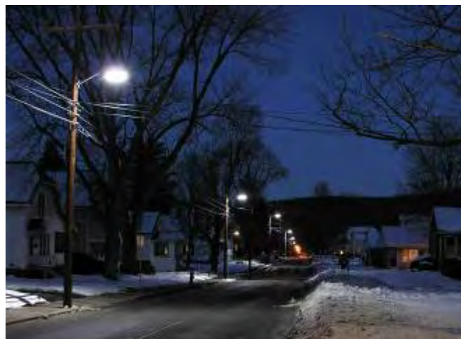
Figure A4-3. Fluorescent lighting with drop lens
