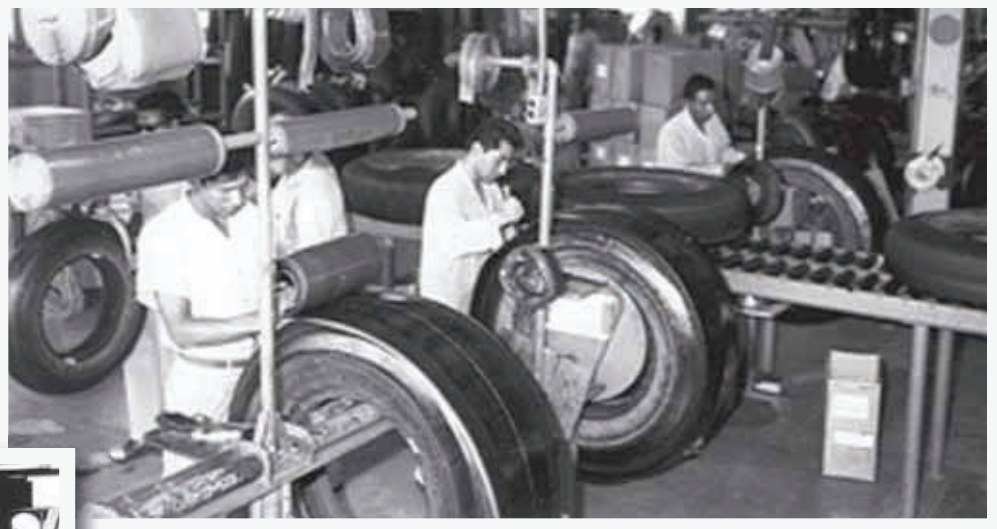
Inmates apply new rubber to tires as part of the reconditioning process at the FPI operation in Texarkana.
