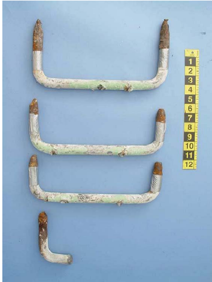
Figure 3. Photograph of U-bolts after removal from barrier.
