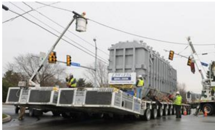
Figure 4. Transport of Large Power Transformers
