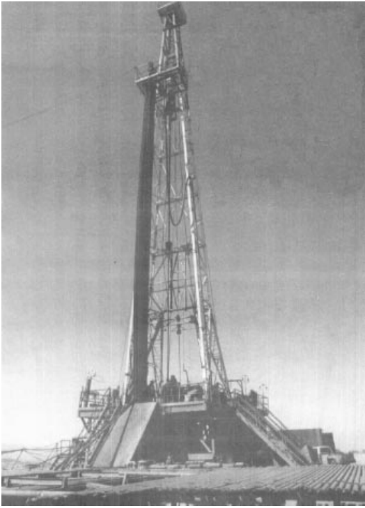
A Stevens Zone rig drills for oil at the Elk Hills Naval Petroleum Reserve in California.
