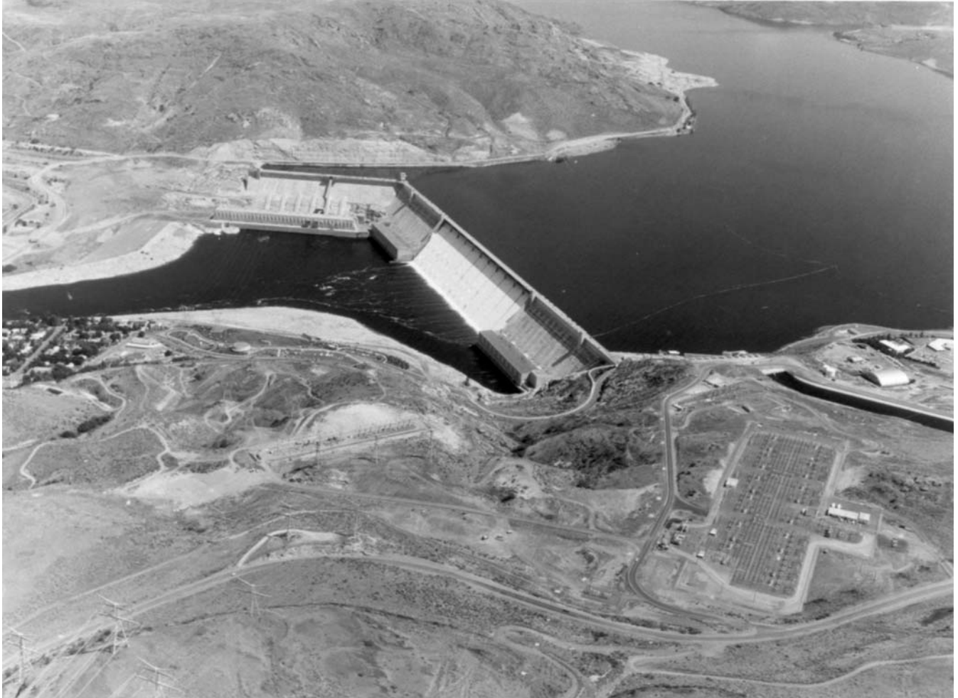
Grand Coulee Dam, Washington State. Source: U.S. Bureau of Reclamation.
