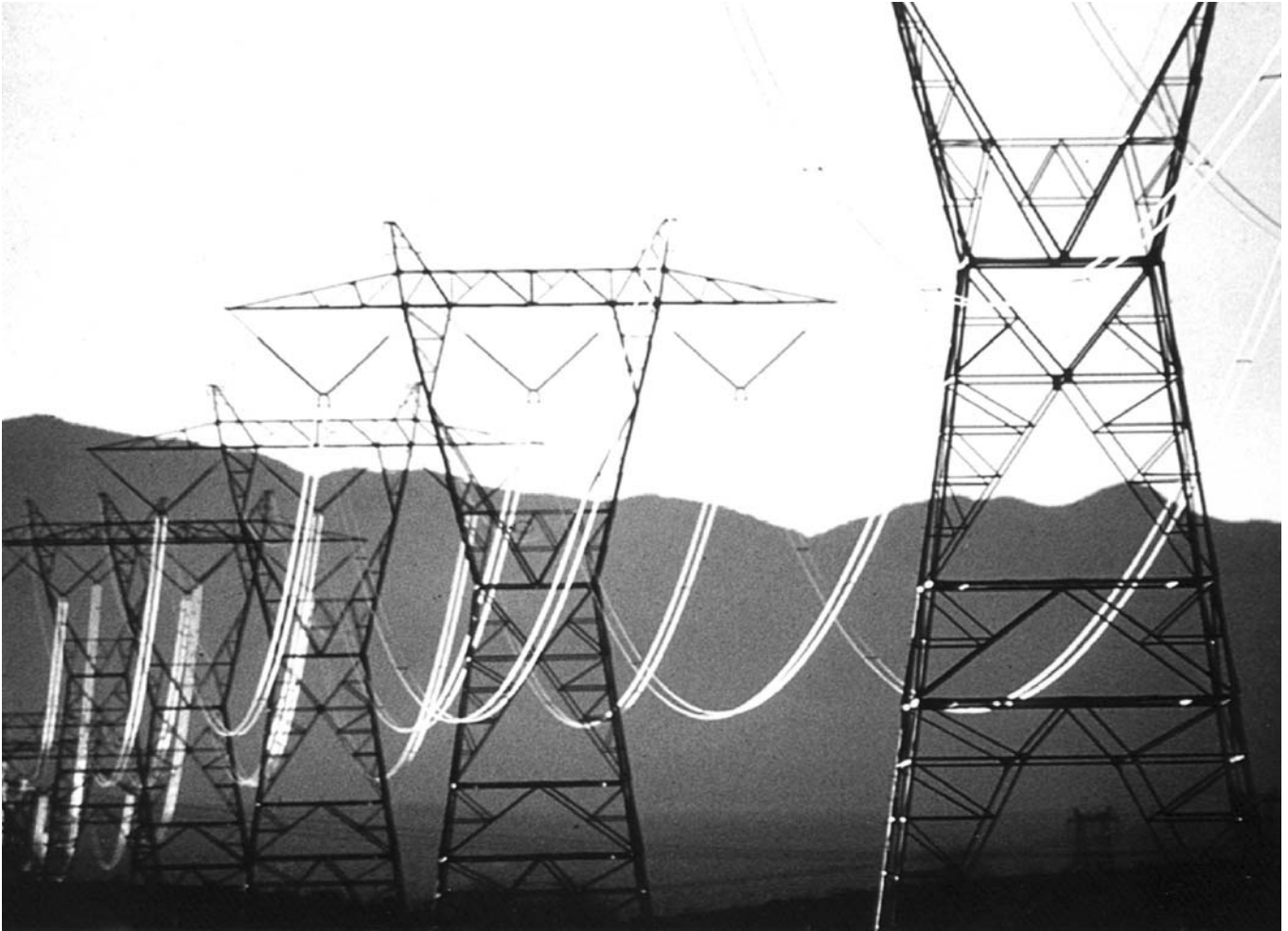
High-tension power lines and towers. Source: U.S. Department of Energy.
