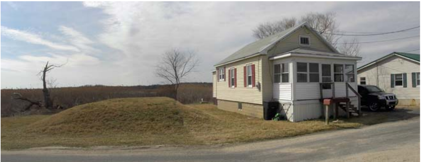
Photo 42. Mounds-based septic system next to house. Along the back side of Pickering Beach, Delaware (March 2009). Photo source: ©James G. Titus, used by permission.
