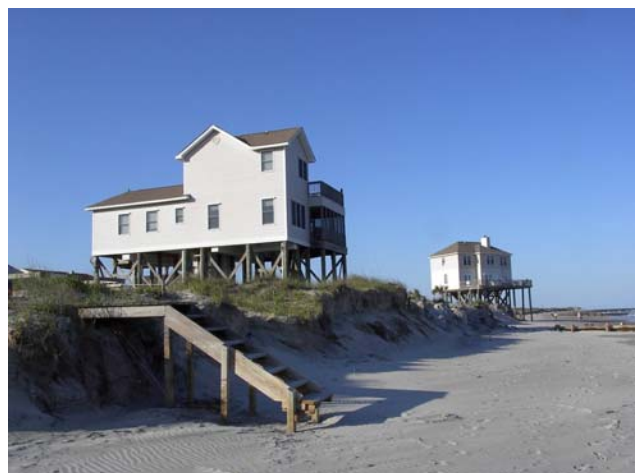
Photos 33 to 35. Most states show flexibility on removal of buildings on the beach as a result of erosion. Top: Westerly, Rhode Island (March 2003). Middle: Kitty Hawk, North Carolina (June 2002). Bottom: Folly Beach, South Carolina (April 2004). Photo source: ©James G. Titus, used by permission.
