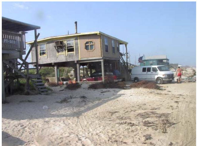
Photos 22 and 23. Two Views of House Encroaching Seaward of the Vegetation Line along the Texas Gulf Coast. Surfside, Texas (May 2003). The beach was the primary means of access. Although these homes were subject to removal orders, the state did not actively seek removal. The homes were destroyed by Hurricane Ike in 2008. Photo source: ©James G. Titus, used by permission.
