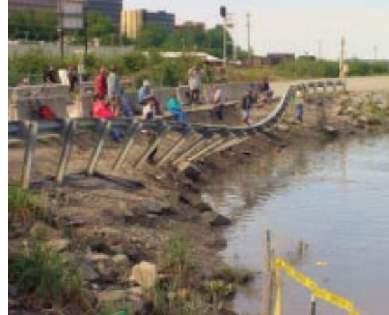
Shoreline restoration of Ship Creek in Anchorage, Alaska.
