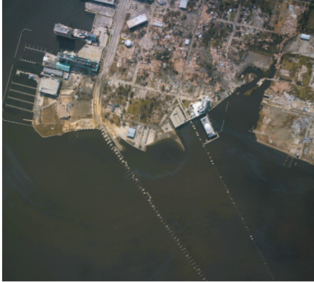
Immediately following Hurricane Katrina, NOS collected more than 10,000 aerial images of the hurricane-damaged areas along the coasts of Alabama, Mississippi, and Louisiana. Photo: National Geodetic Survey
