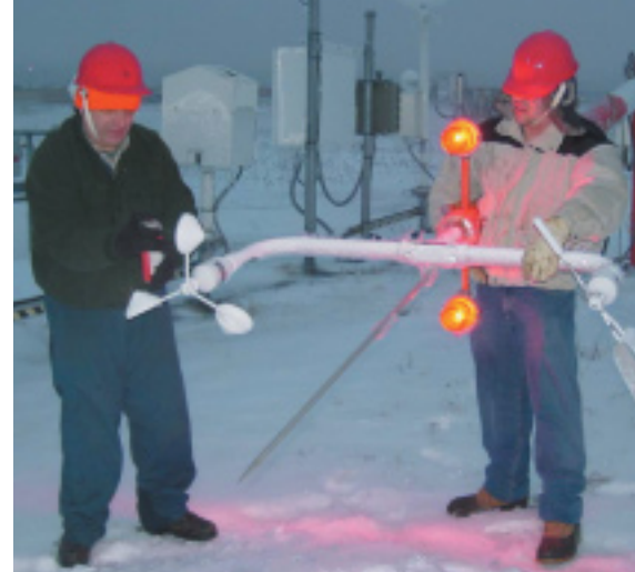
Electronic Technician Martin Lee (left) and Electronic Systems Analyst Don Price of the Weather Forecast Office in Duluth, Minnesota, de-ice Automated Surface Observing System equipment. A December 2004 ice storm left nearly an inch-thick coating of ice on the wind equipment. Photo: Ed Shimon, NWS
