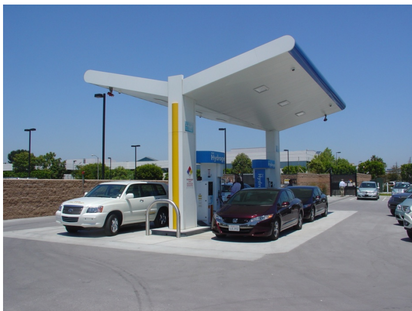
Figure 3.6.4 Fueling station using pipeline hydrogen - If a hydrogen pipeline is located nearby, the cost of building the hydrogen production system can be avoided, lowering the cost of dispensed hydrogen (photo source: NREL).
