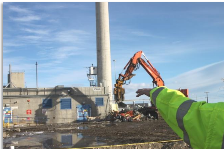
Demolition of PFP's 2736-ZB Vault Complex continues
