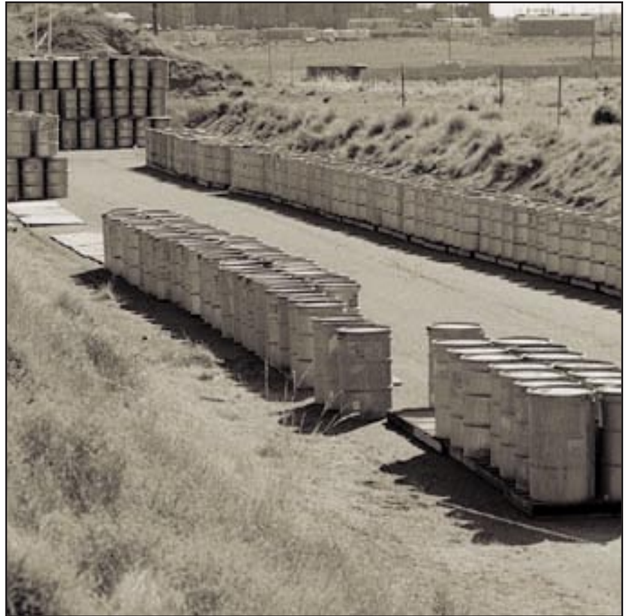
Uncovered drums of transuranic waste in this large trench are among the first to be retrieved more than a year early. The current schedule calls for retrieving 10,000 drums by 2004.
