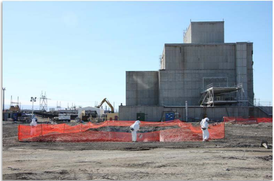
115KE building demolition
