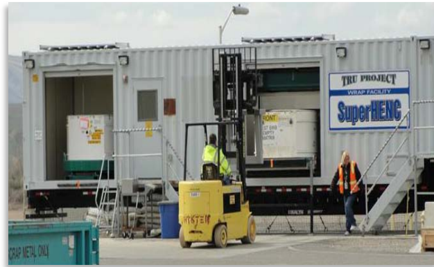
Loading waste box
