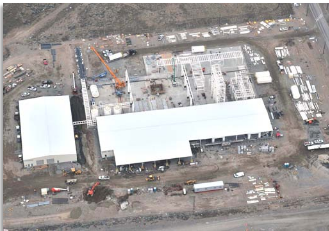
Aerial view of 200 West Groundwater Treatment Facility
