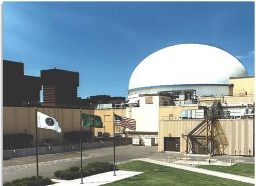
Fast Flux Test Facility
