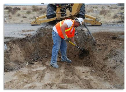
A worker helps create the site for a road crossing. Over 100 road crossings are being constructed to protect the high-density polyethylene piping from the weight of heavy vehicles as the pipe crosses under the road in its 42-mile span to connect the DX facility to wells in the 100-HR-3 area.
