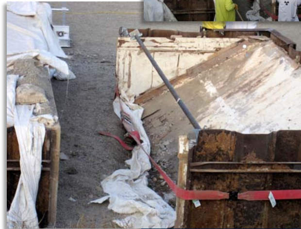
3A Trench 17 Box 82 Sheet Piling and Bracing Installation
