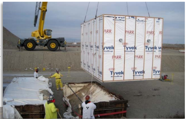
3A Trench 17 Box 82 Wooden Cover Installation
