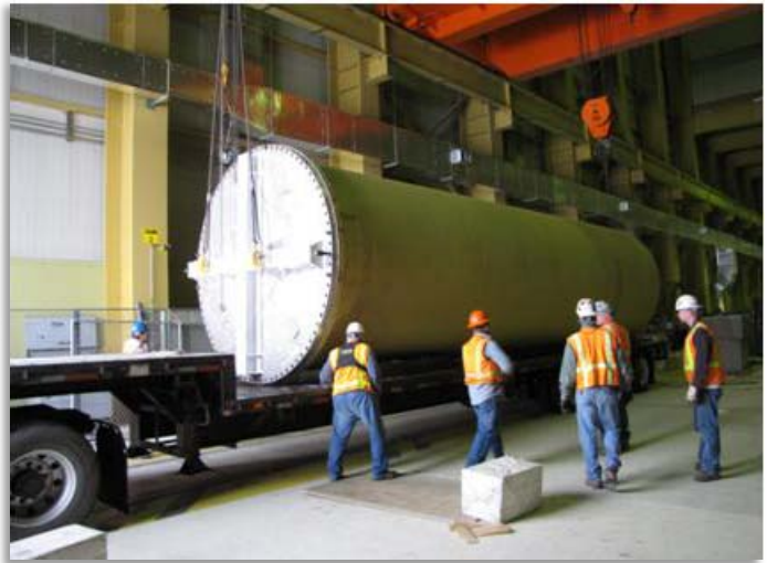
Maintenance and Storage Facility (MASF) Tank Removed
