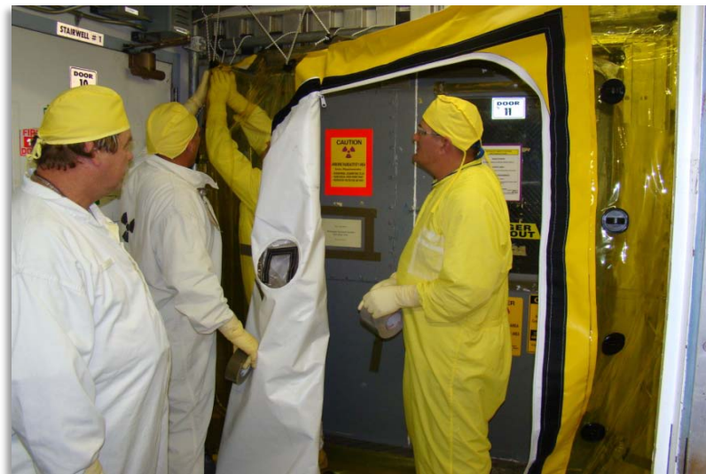
242-Z Team Setting Up the Containment Tent for Sampling of the Tank Room Atmosphere
