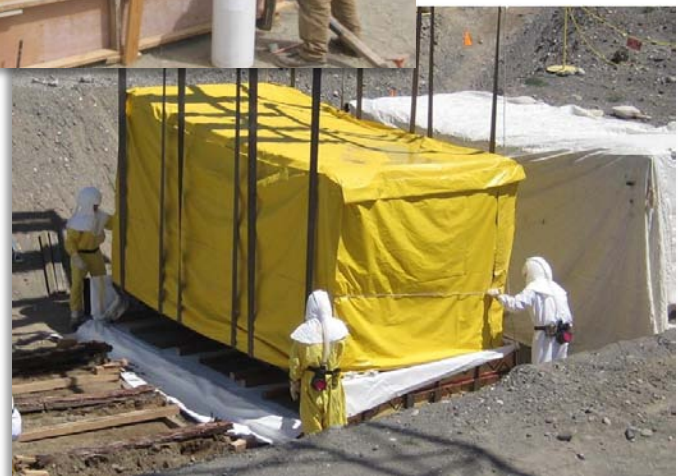
Fiberglass- reinforced plywood box of suspect TRU waste that has deteriorated after years in underground storage
