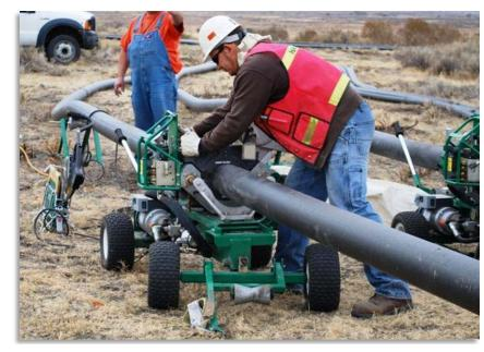
A worker bonds two pieces of high-density polyethylene (HDPE) piping. Over 42 miles of HDPE piping is being installed to connect the DX groundwater treatment facility to wells in the 100-HR-3 area.
