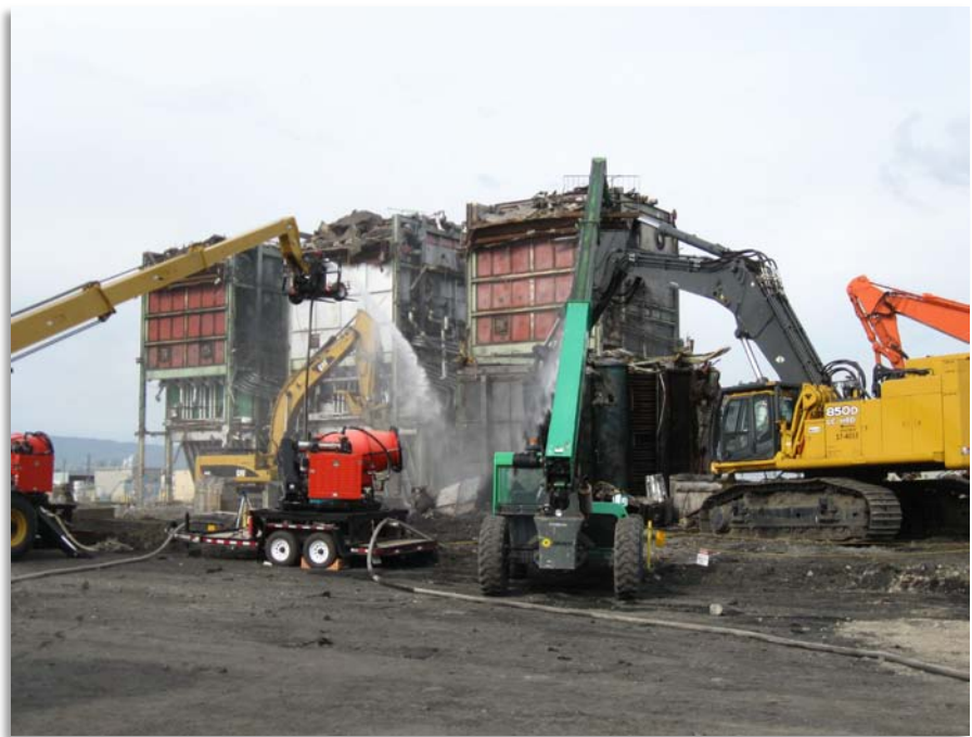
Demolition of 284E Boiler
