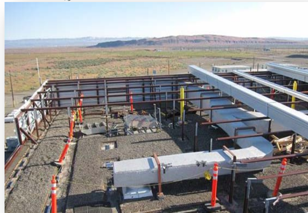
WESF Upper Roof Upgrades
