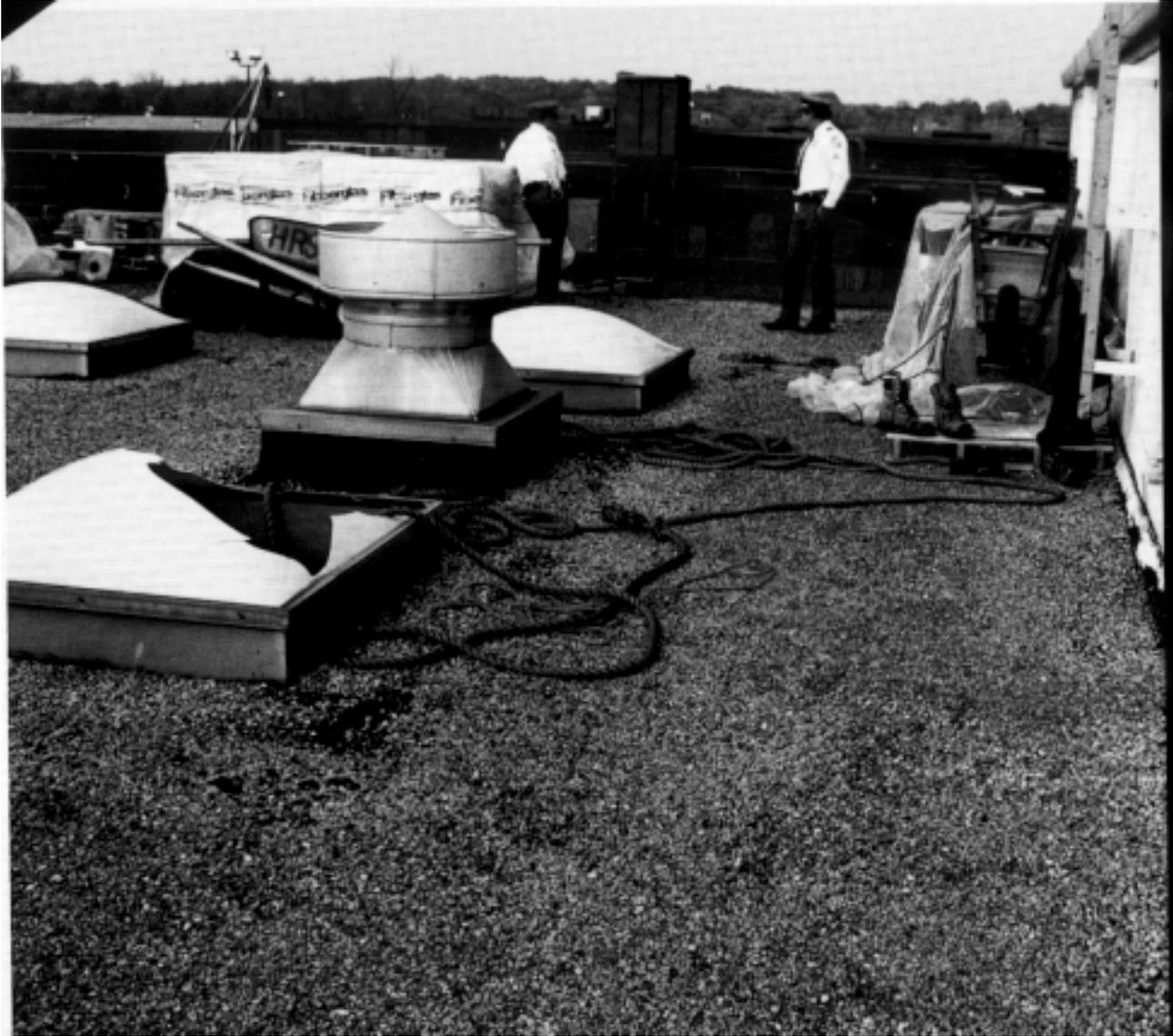
*Figure 2. This Figure Shows an Intact Smoke Dome Type Skylight Just Opposite the Broken Skylight. The Fixed Ladder Providing Access to Roof of the Higher Section of the Building is Shown at Left.*
