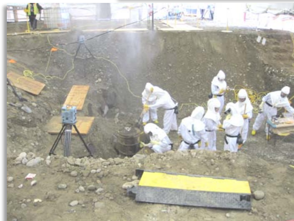
12B Trench 17 Drum Removal
