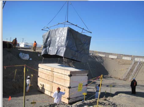
3A Trench 17 Box 14 Excavation and Preparation for Removal
