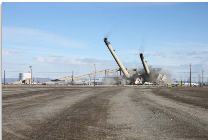
Demolition of the 284-W stacks
