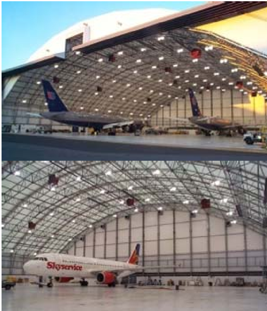
Figure 6-1. Example Rubb® Structure (255-Foot Span by 270 Feet Long).
