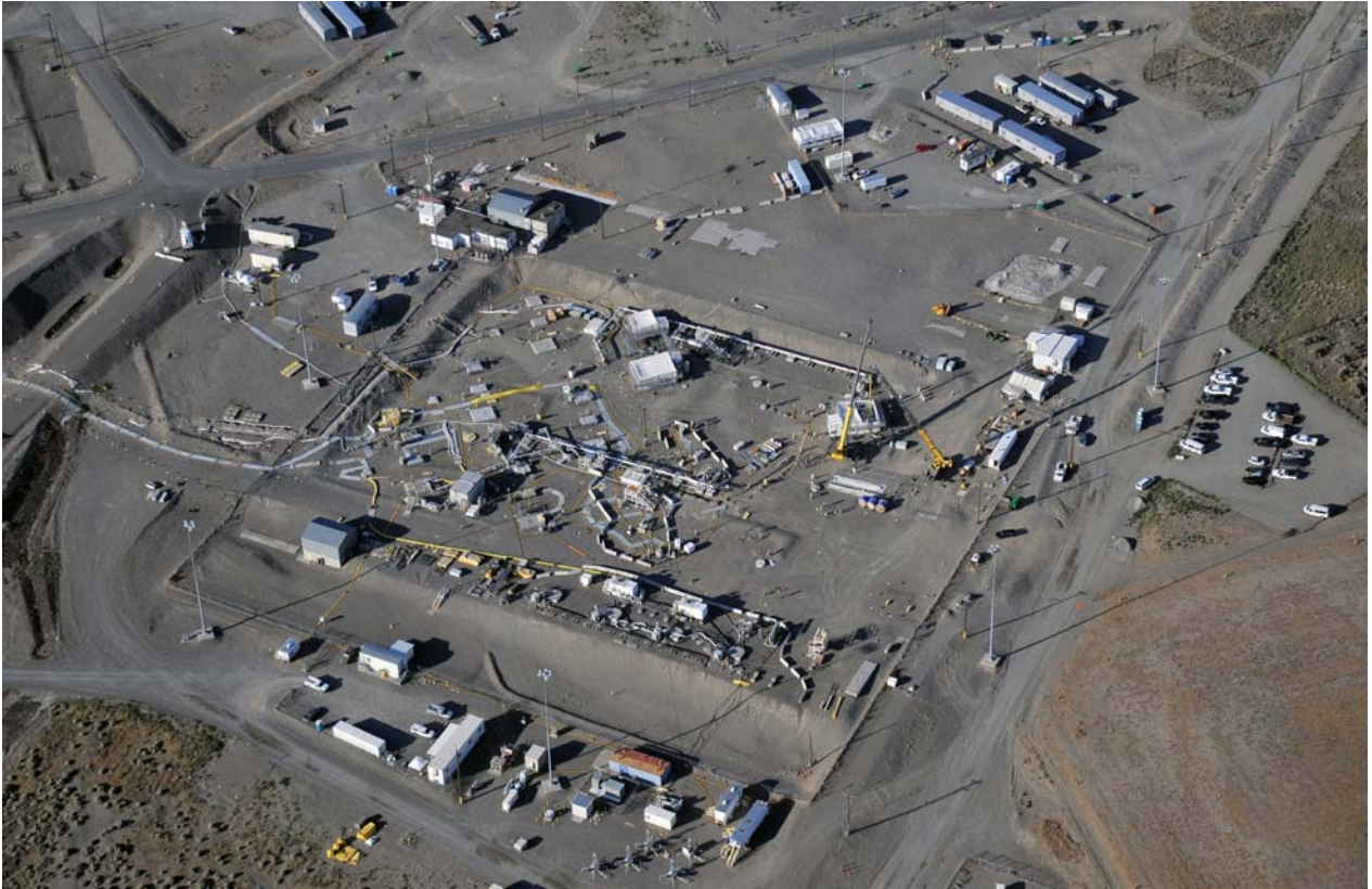
Figure 4-1. 241-C Tank Farm Aerial (2008).
