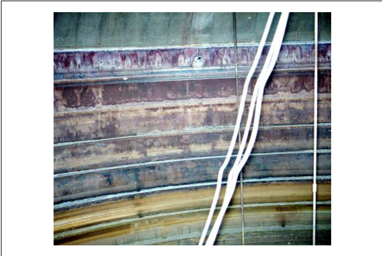
Figure 4-2. Tank SX-110 Interior Wall (February 20, 1987)
