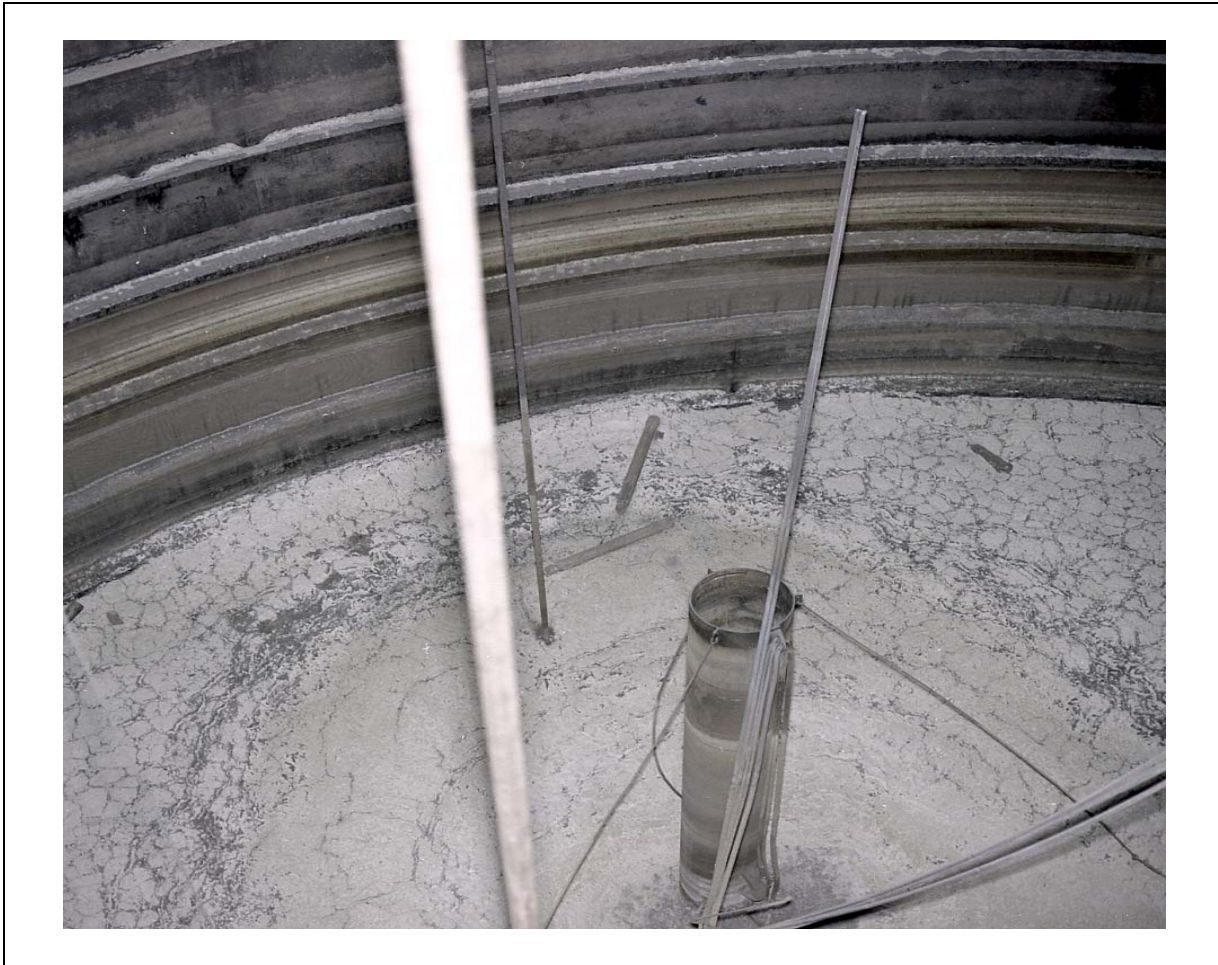
Figure 3-3. Tank 241-SX-110 Dry Waste Surface, June, 1982. The polyethylene shipping bottles can be seen scattered on the waste surface.
