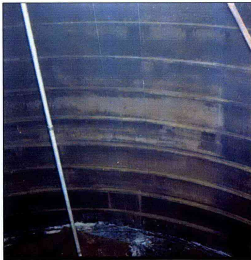
. Figure 3-4 Torn and Buckled Liner in Tank A-105
