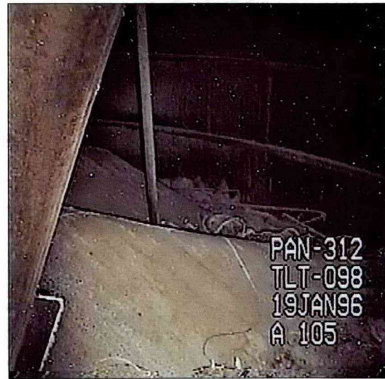
. Figure 3-4 Torn and Buckled Liner in Tank A-105
