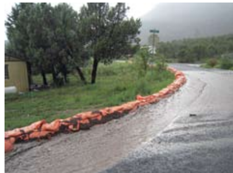
Runoff on Locust Ave.
