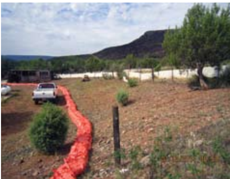
K-Rails and sandbags designed to direct flow
