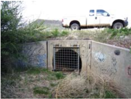
Major drain under highway
