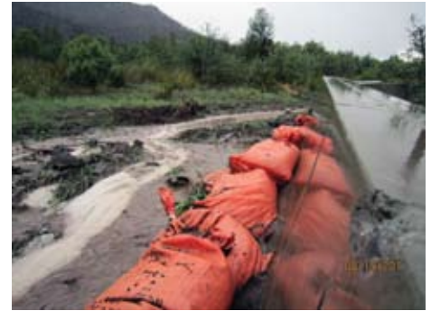
Flow channeled along sandbags and K-rails
