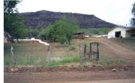
K-rails and sandbags installed to protect homes
