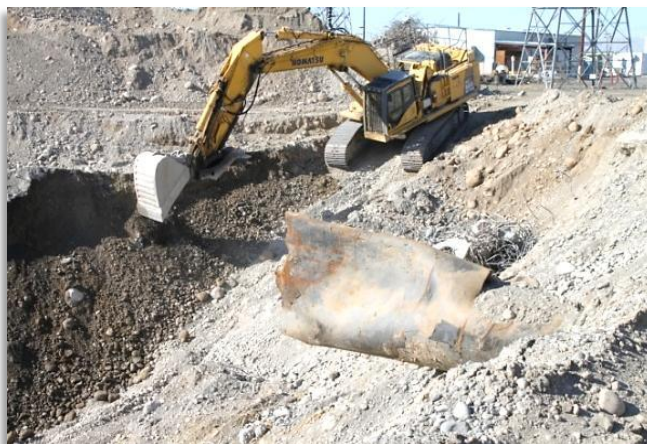
Demolition continues on the substructure of the former 182K building.
