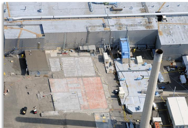
Previous location of the 2736-ZB Vault Complex at PFP
