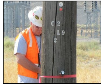
Inspecting Central Plateau High Voltage Distribution System wood poles.
