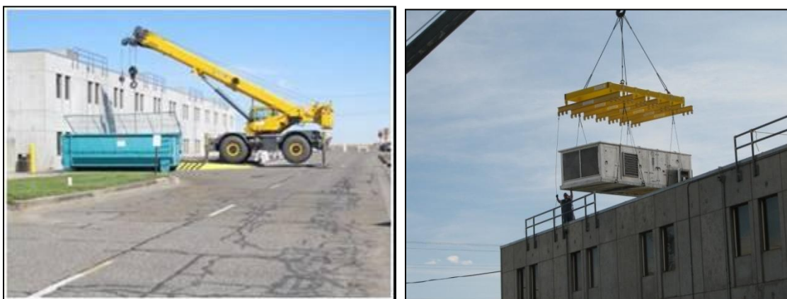
Crane & Rigging supports replacing HVAC units at 2750E
