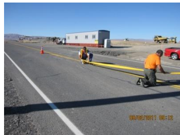
Installing temporary yellow tape on Route 3
