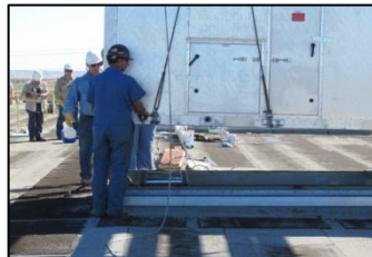
HVAC install at 2750E
