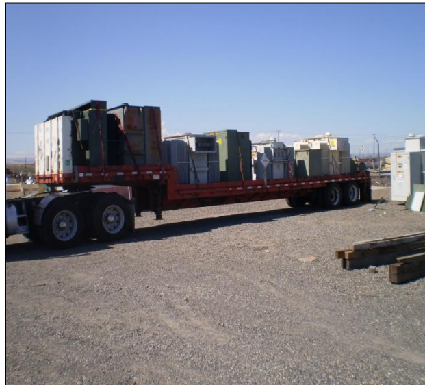
Excess transformers are loaded onto a low-boy trailer and ready to be shipped to Clean Harbors
