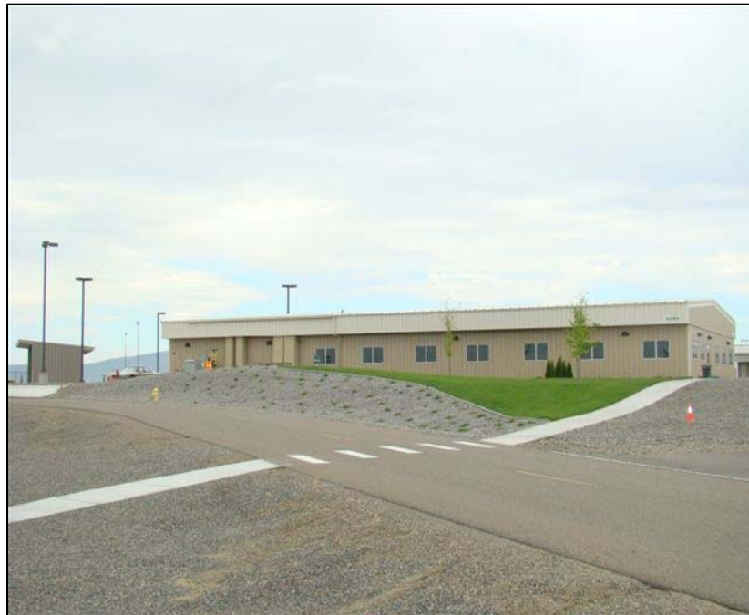
Project T-221, "Completed Hammer Operations Building"
