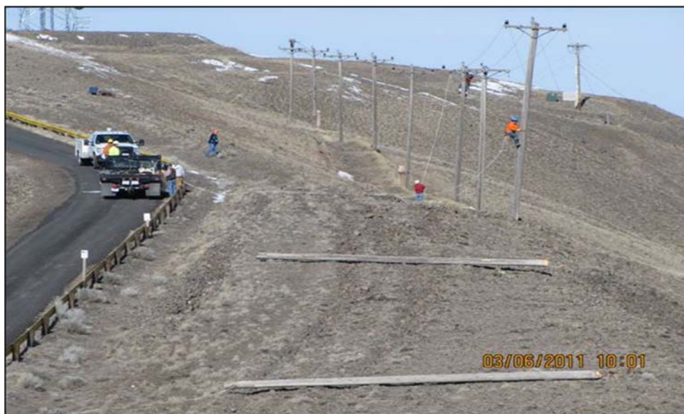
Rattlesnake Mountain pole removal activities
