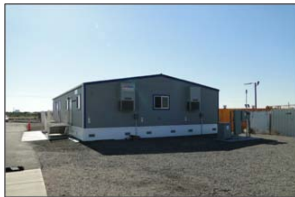
Project L-750, Completed Crane & Rigging Triple Wide Trailer
