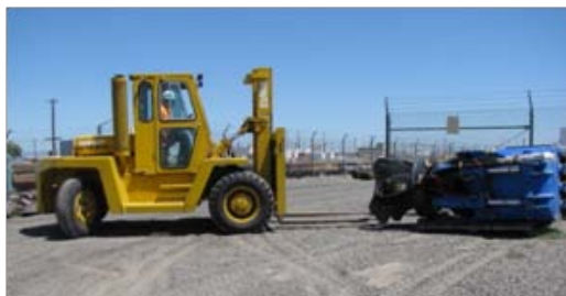
Clamshell bucket hauled via flatbed to the 200 East Area
