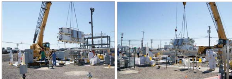
Exhauster removal at AW Farm
