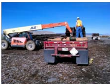
Transporting railroad ties from the 100 B&C Areas
