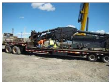
Teamsters securing John Deere excavator attachment
