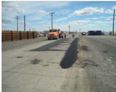
Road repairs at 222S responding to a safety concern
