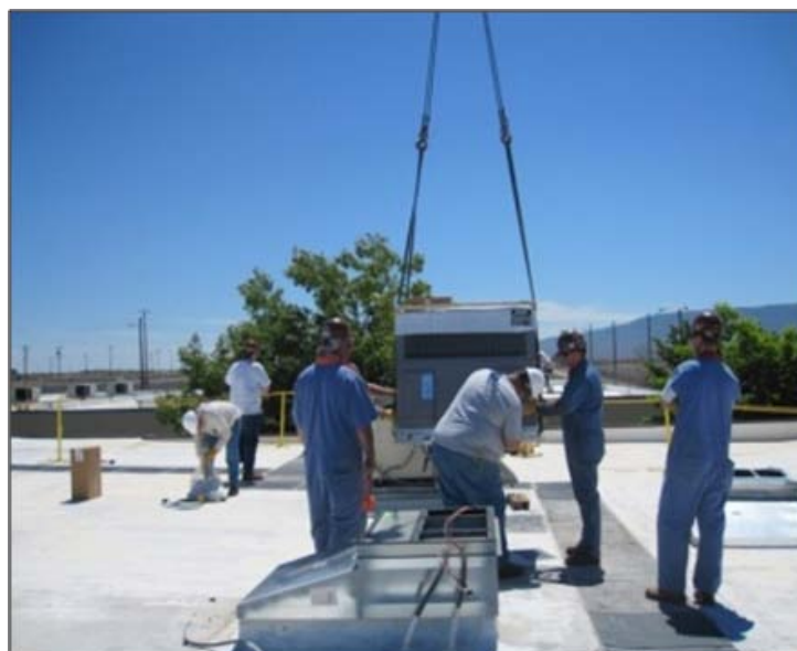
Completing the installation of HVAC units for WRPS at 2752E facility
