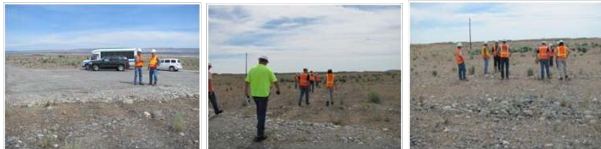
Test Trench excavation walk down
