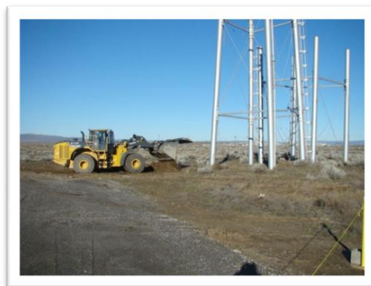
Leveling ground for D&D of the REDOX water tower
