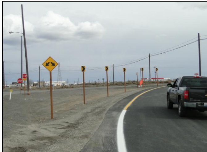
Newly paved Route 3/Route 4 turning lane
