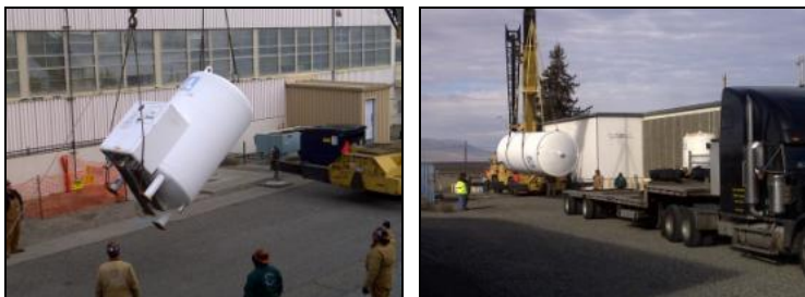
Removal of the liquid nitrogen tanks in the 300 Area
