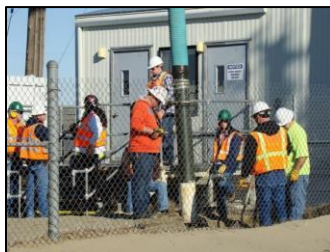
Blow Sand Removal at T-Farm using the Guzzler
