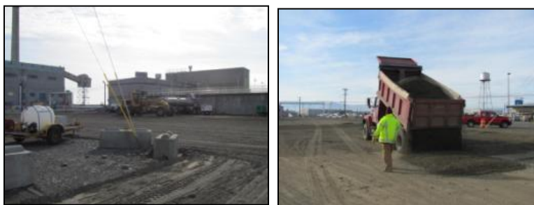
Parking lot repairs at MO-2209
