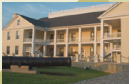
St. Francis Barracks in St. Augustine FL has served as headquarters for the Florida National Guard since 1907. Photo by Chris West
