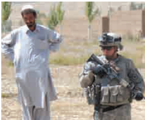
SGT George W. Brimer watches as team members perform a quality-assurance inspection of a cool-storage facility being built in the Ahmedabad district of Afghanistan's Paktia province.
