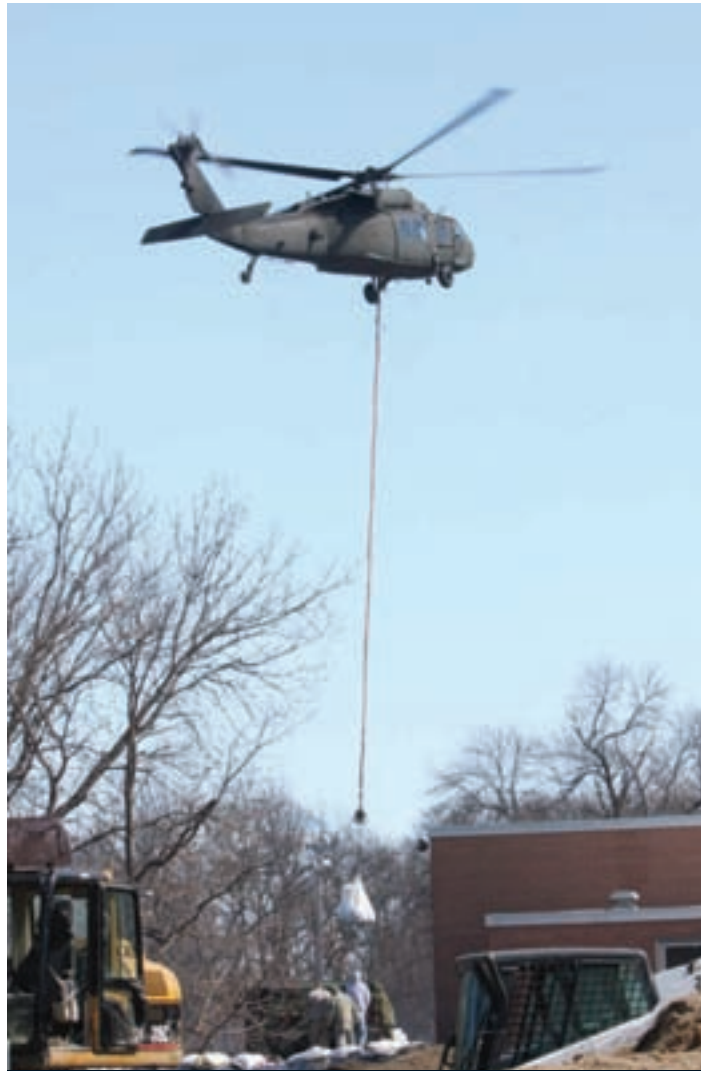
ONE-TIME USE BASKET An ARNG Black Hawk helicopter places a one-ton sand basket on a levee near the Oak Grove Lutheran School in downtown Fargo.
