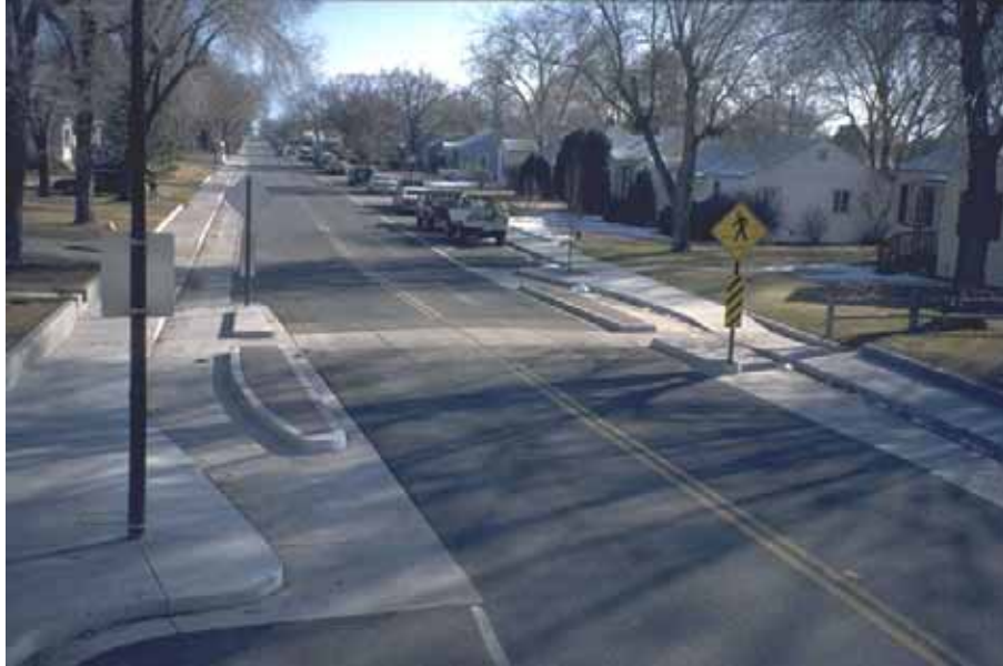
Figure 20-6. Photo. Where possible, cyclists should be provided with cycle slips that enable them to bypass speed humps.
