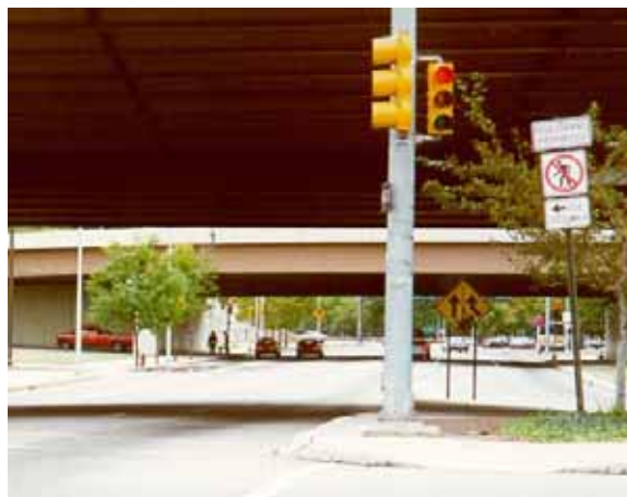
Figure 10-3. Photo. Pedestrians are restricted from continuing straight and are encouraged to cross left to avoid a traffic merge lane.
