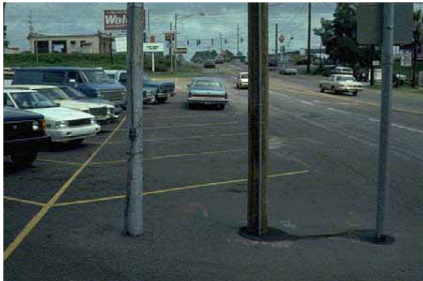
Figure 7-2. Photo. Parked cars and a lack of sidewalks along the road's edge create unsafe conditions for bicyclists and pedestrians.
