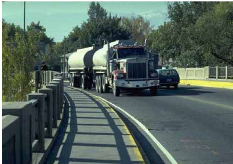
Figure 22-2. Photo. Bridges are a recurring theme in many tort liability claims.
