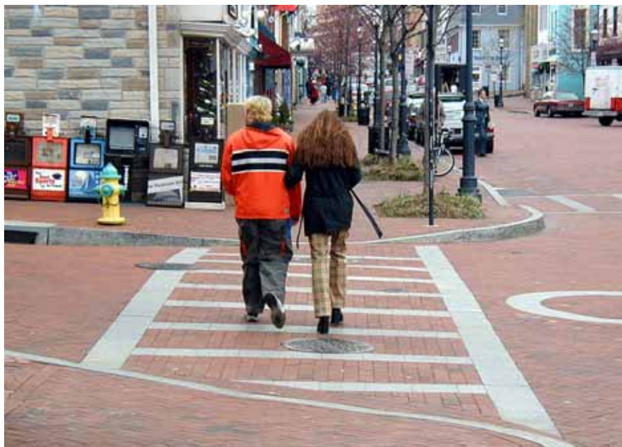
Figure 3-20. Photo. A crosswalk can increase the visibility of a pedestrian path.
