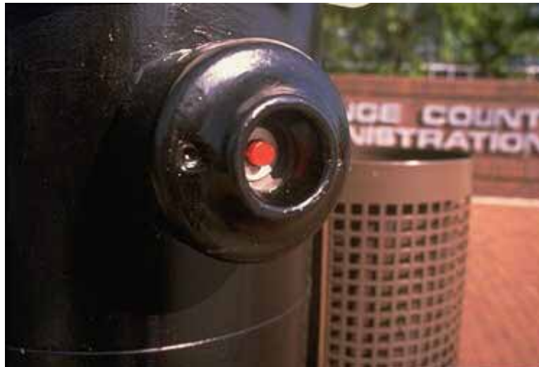
Figure 11-12. Photo. Example of obscure pedestrian pushbuttons; pushbuttons should be conveniently placed and clear from obstacles.
