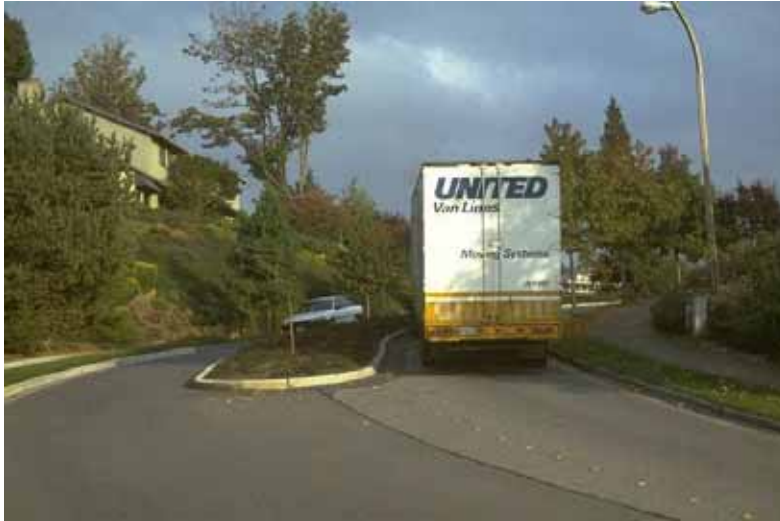
Figure 20-12. Photo. This traffic-calming measure uses a landscaped median to narrow the travel lanes.
