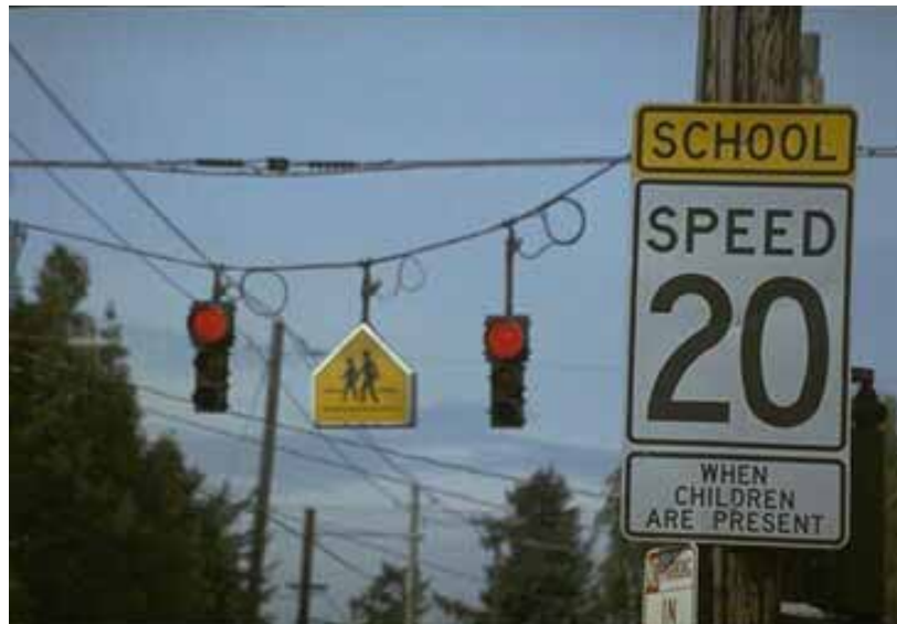
Figure 10-6. Photo. Flashing lights, school crossing signs, and a low speed limit gives motorists plenty of warning of the crossing area ahead.
