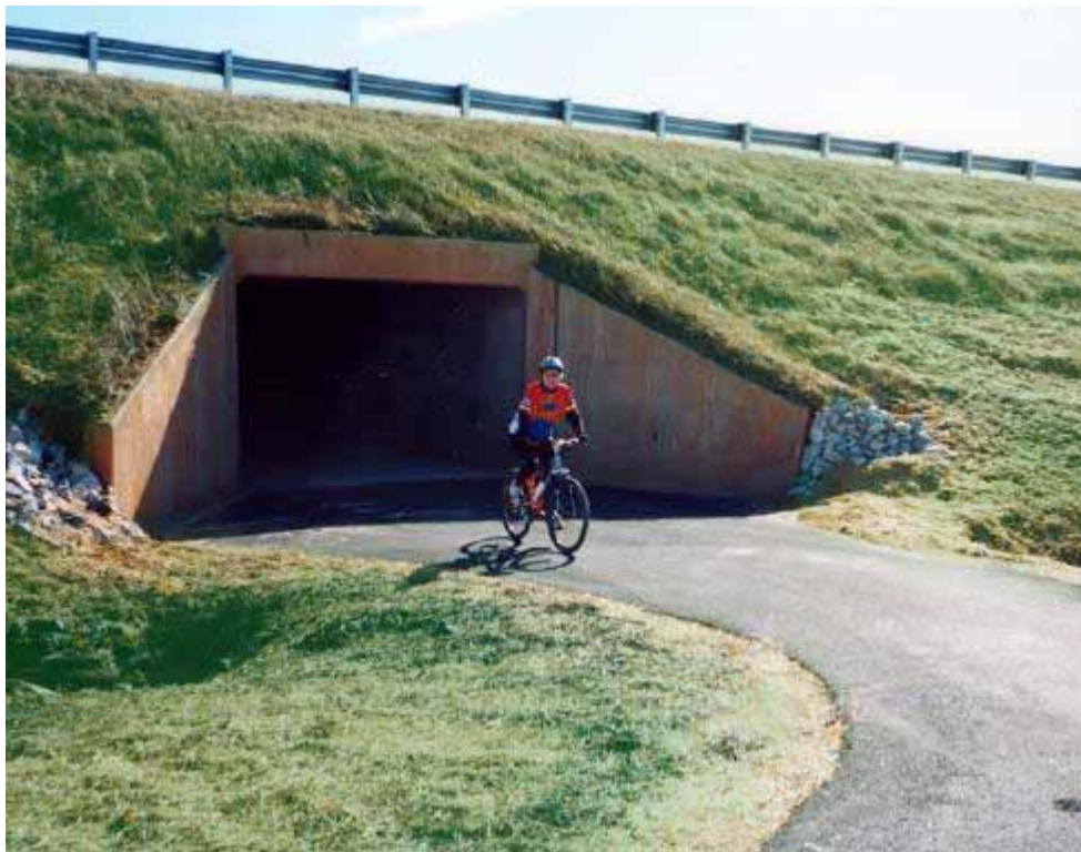
Figure 12-9. Photo. An underpass continues this shared-use bicycle path beneath a four-lane highway with high traffic volume.
