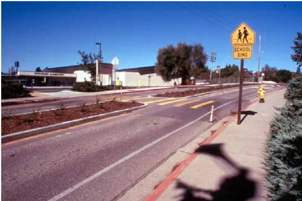
Figure 10-1. Photo. The sign and crosswalk markings at this midblock crossing alert drivers to pedestrians going to school.
