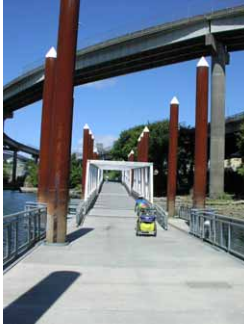
Figure 19-8. Photo. Bridges and floating sections allow paths to cross water and maintain continuity (Eastside Esplanade, Portland, OR).
