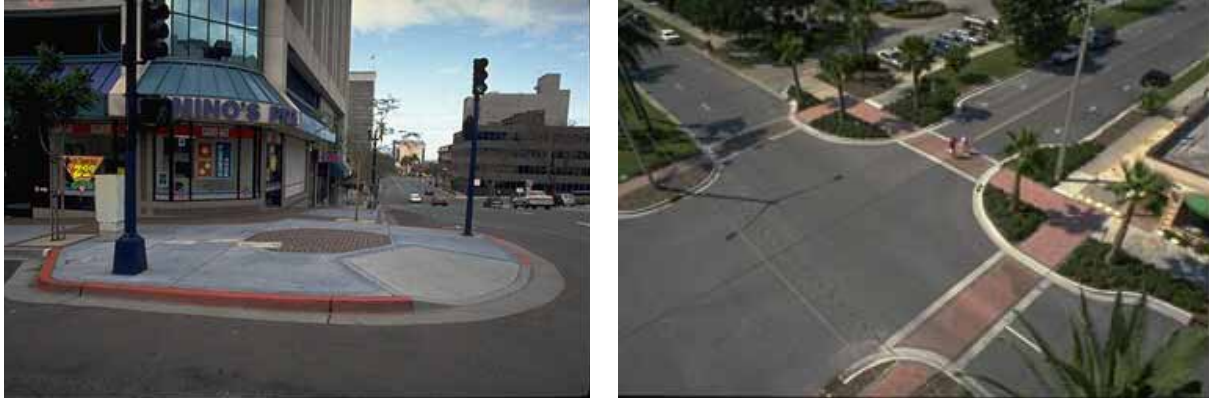
Figure 11-10. Photos. Curb extensions reduce crossing distances for pedestrians and provide additional corner storage space.
