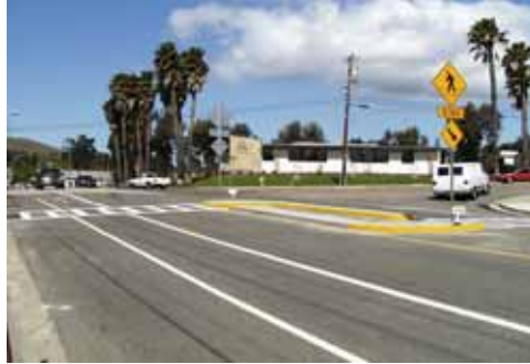
Figure 11-8. Photo. Staggered pedestrian crossings (Z-crossings) treatment in San Luis Obispo, CA.
