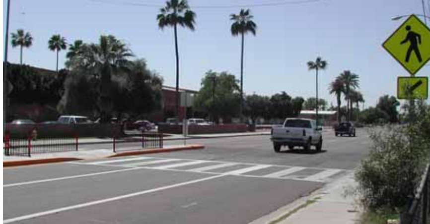
Figure 20-9. Photo. This median refuge island provides railing and a staggered crossing area to direct pedestrian views toward oncoming traffic.
