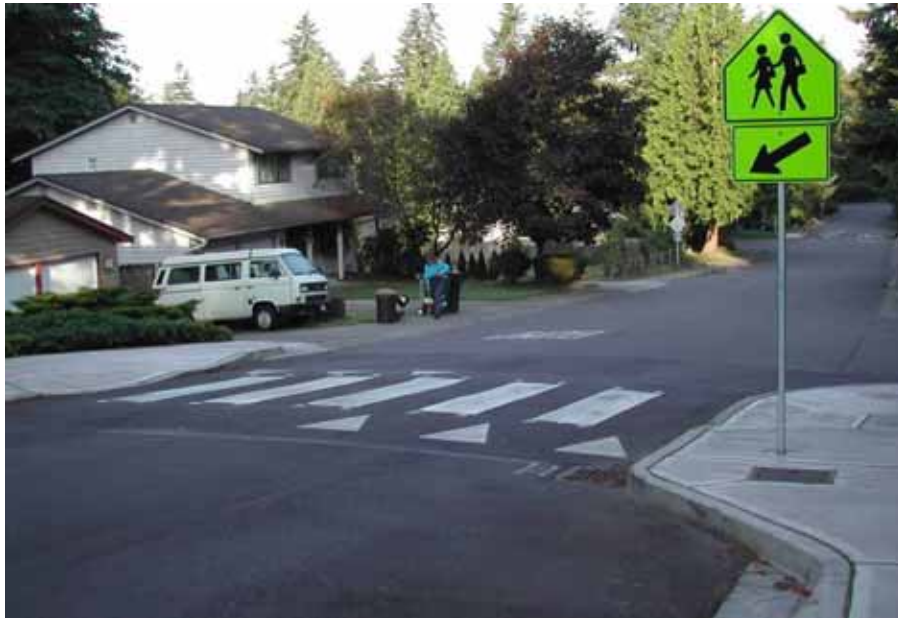
Figure 20-5. Photo. Speed humps can be combined with curb extensions and a winding street alignment.
