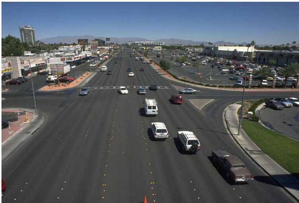
Figure 1-1. Photo. Wide suburban streets like this one were not built to accommodate or encourage walking.
