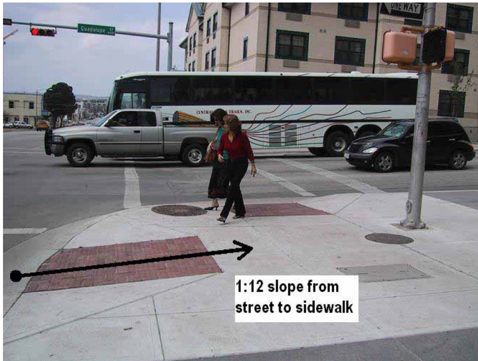
Figure 8-15. Photo. Perpendicular curb ramp.
