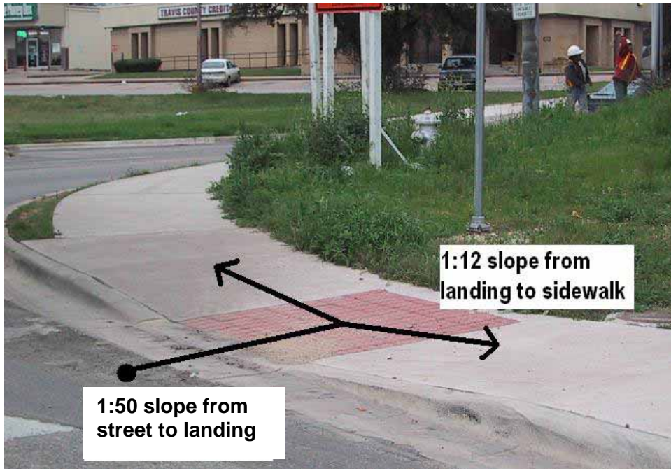
Figure 8-16. Photo. Parallel curb ramp.
