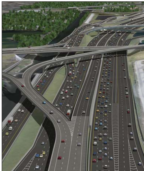
I-595 corridor roadway improvements
