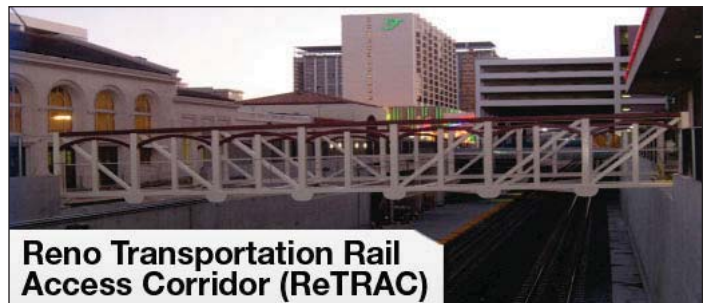
The ReTRAC project used several innovative revenue sources, including revenue from a special downtown assessment district, to repay financing.
