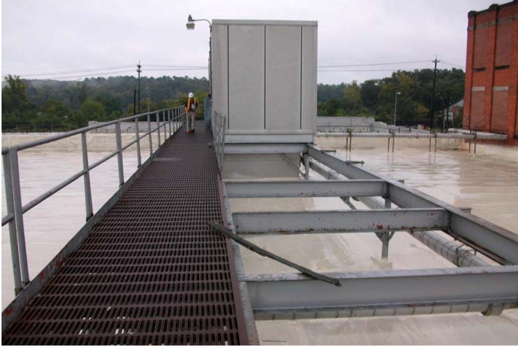
Photograph No. 9: Metal walkway grating and associated handrails of the rooftop air handling unit above Weave Room No. 2.
