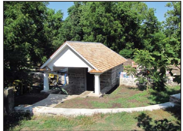
The Springhouse on the Saline Courthouse National Park property during redevelopment.
